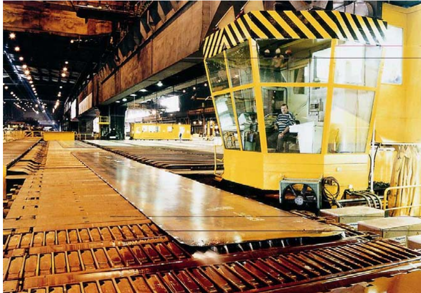
Fig 8.3.1: Total view of the testing system within the roller conveyor
