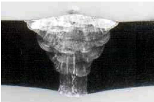
Figure 4 Gas Tungsten Arc Welding ( 141 -GTAW)
