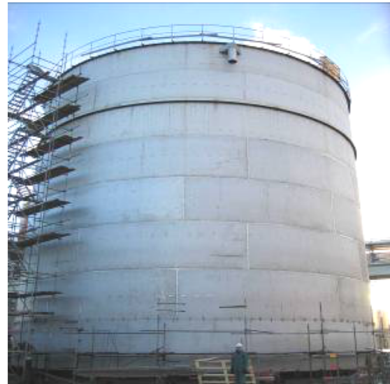
Sweden, storage tank 2304 grade
