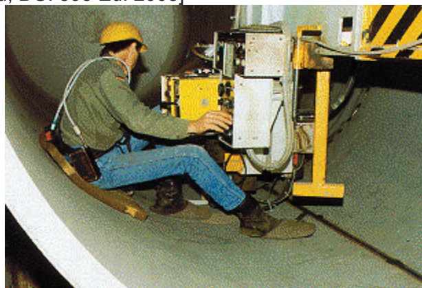
Figure 10-3: Submerged arc welding with low emission of hazardous substances [Source: Spiegel-Ciobanu, BGI 593 Ed. 2008]
