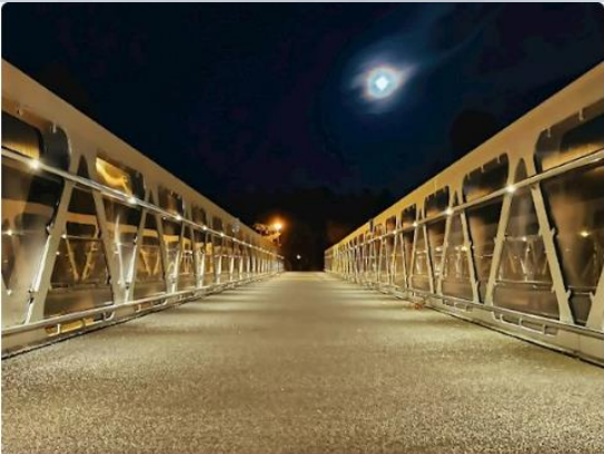
Welding of stainless steel bridges
